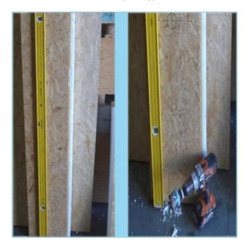
Another core is drilled at the service entry locations. Insert your catching device into the bottom hole so the hot ball is collected and does not continue down the panel, also the ball is hot, DO NOT catch it in your hands as it will burn you.
